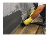
**1.** • Apply a first coat of VANDEX BB 75 E (3 kg/m², 1.5 mm, mixing instructions as per Data Sheet VANDEX BB 75 E), at least 1 cm beyond the VANDEX CONSTRUCTION JOINT TAPE.
