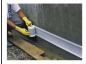
**3.** Overcoat VANDEX CONSTRUCTION JOINT TAPE with a second coat of VANDEX BB 75 E (2 kg/m², 1 mm) and smooth the surface with damp brush.
