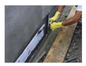
2. Immediately place the VANDEX CONSTRUCTION JOINT TAPE in the freshly applied VANDEX BB 75 E coat. Then, embed both fabric edges in the VANDEX BB 75 E
